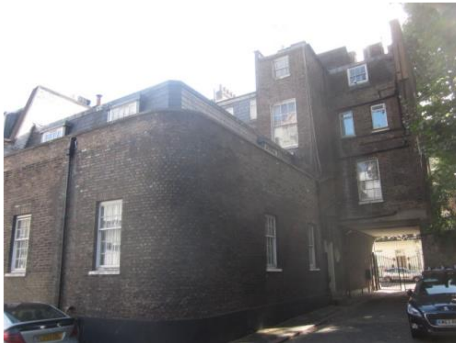
Rear wing from within Albion Close.
